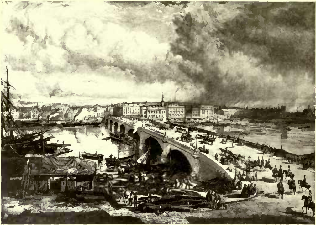
FIG. 418. Broomielaw Bridge, 1850. From Water Colour by Sam Bough, R.S.A.
