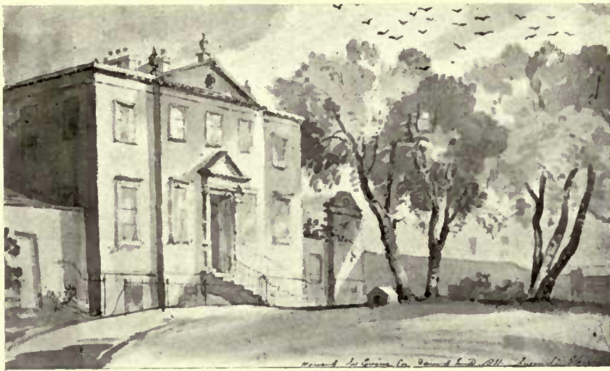
FIG. 416. House of James Ewing, Dean of Guild, 1831, on site now occupied by the Queen Street Station of the North British Railway.
