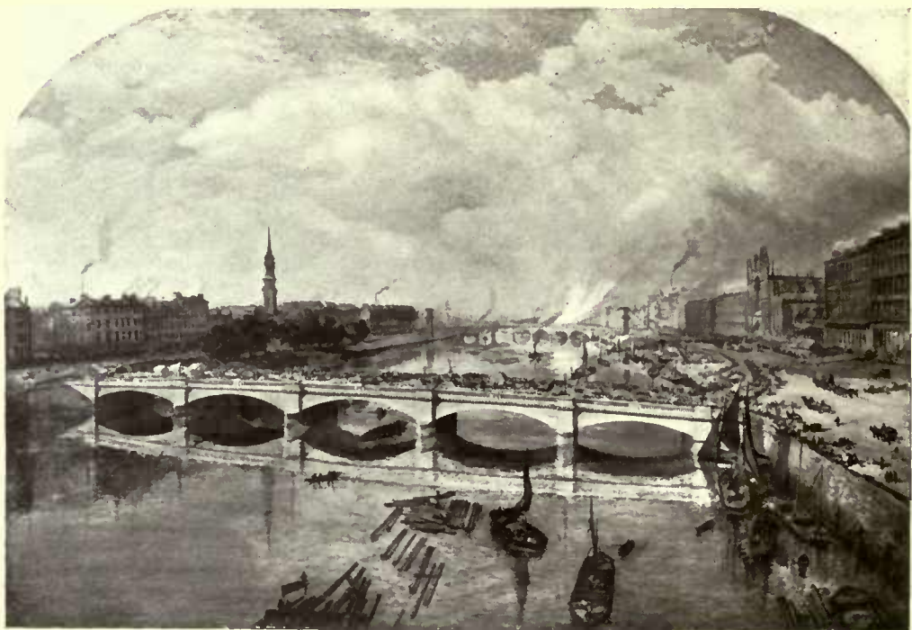
FIG. 419. Stockwell Bridge, 1853. From Water Colour by Sam Bough, R.S.A.
